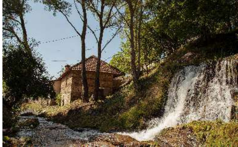
Figure 9 – Waterfall overflow from the channel powering the recently restored mill. Photo: Rand Eppich
