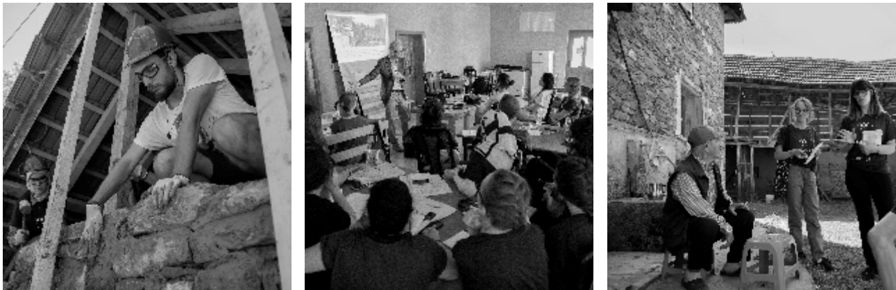
Figure 34 – The Heritage Lab Workshop combined practical field work in conservation, international expertise with local knowledge obtained through interviews. Photo: OSCE/CHwB Dardan Rushiti
