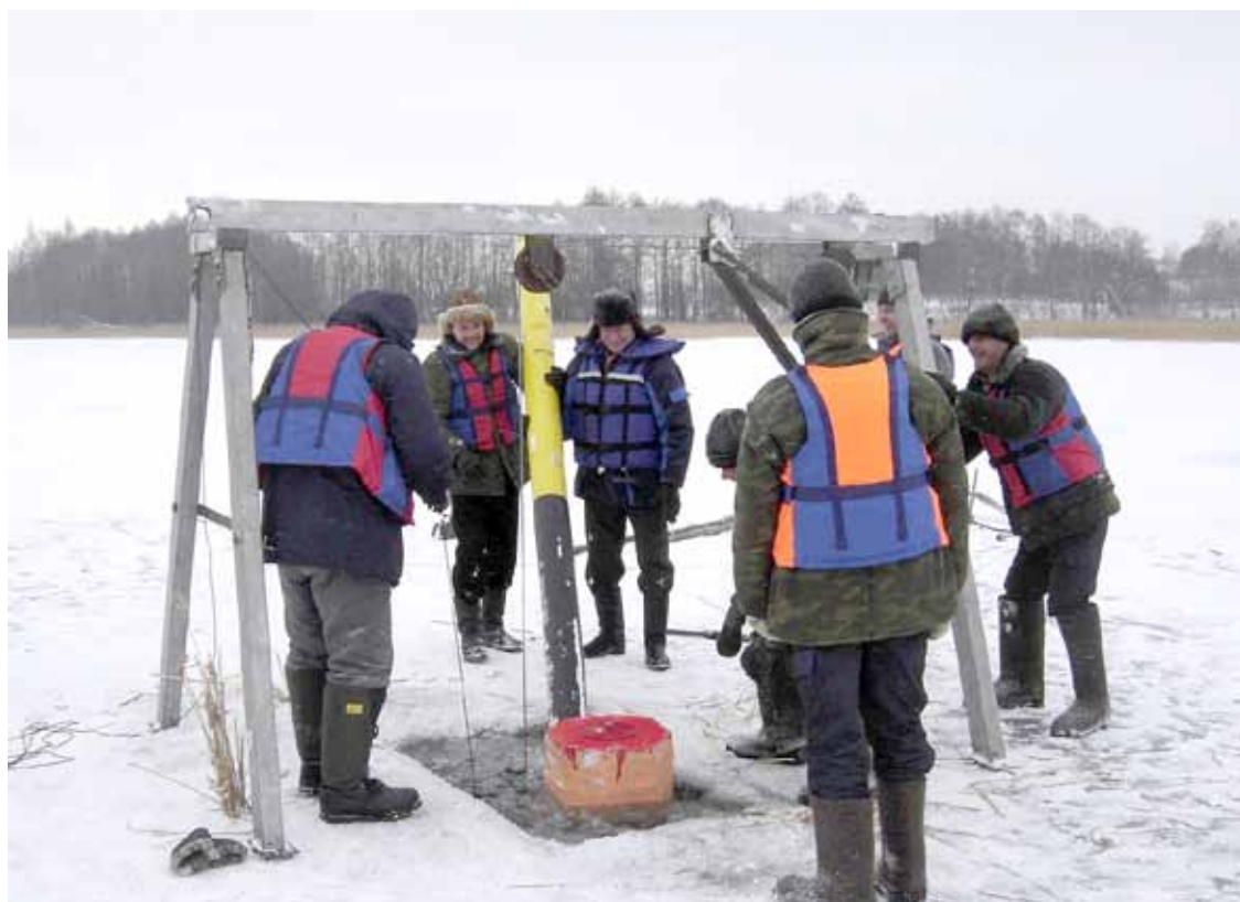
Fig.36. Emplacing a lake boundary marker (a buoy) with a float.
