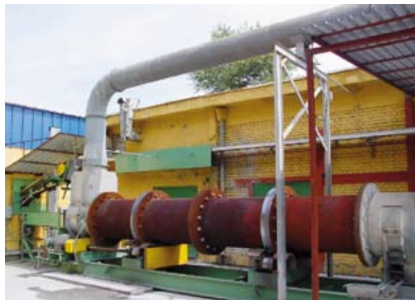
Figure 4.1: Outside view of a rotary kiln furnace (courtesy NAMSA)
