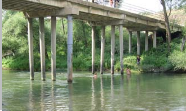
THE BRIDGE AREA FOLLOWING THE CLEARING OPERATION
