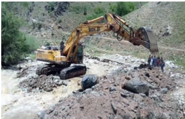
Bank reinforcement works in Darvoz district of GBAO
