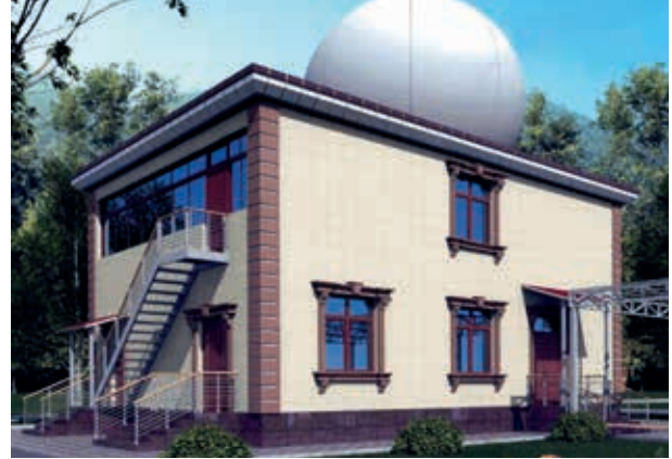
Hail Control Service building after renovation
