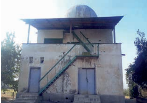
The current condition of the Hail Control Service building
